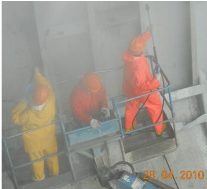
Hold cleaning using HP Washer
