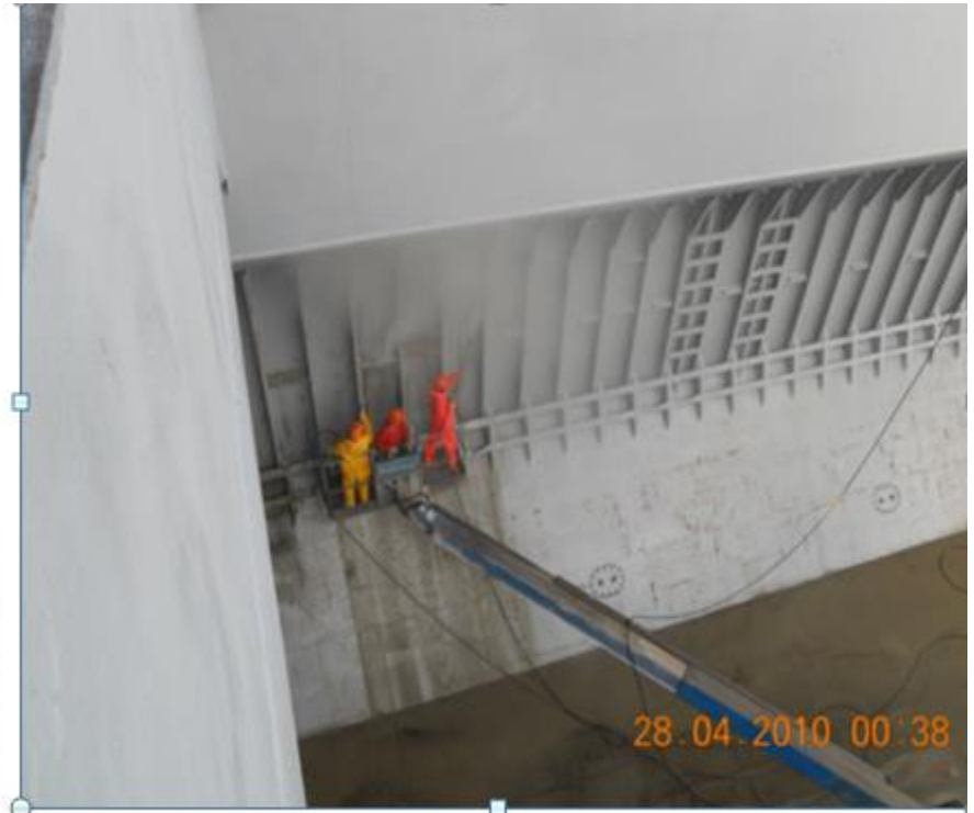
HP fresh water washing
